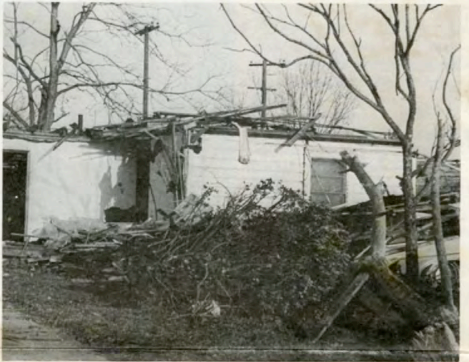
One of the many homes and buildings damaged or destroyed by the Dec. 3 tornado that struck Bossier City.
