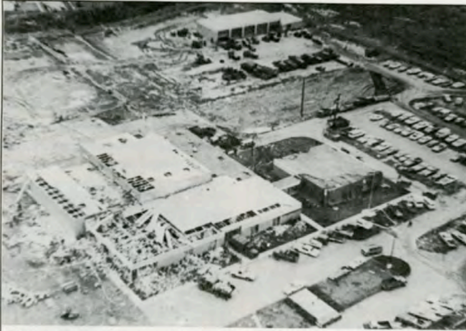
December 3 twister wrecked a large portion of new Bossier City Armory.
