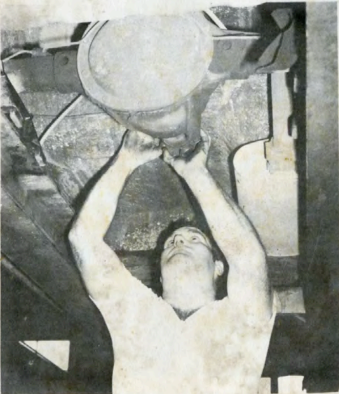
Maintenance teams work thru the day And into the night. . .
