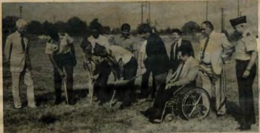
GROUND BREAKING — (From Left to Right) Gene Glanker - Architect; 1Lt. James Boutte - Company Cdr. of 2228th Engr Co.; Steve Shepard - City Council member; SGM Earl Picard - Company SGM of Battalion; LTC Don Bringol - 2228th Engr. Bn.; Don Meeker - City Councilman; Mayor Fred Feeney; Bruce Conlon - City Councilman; Senator John Saunders; Lee Thevenot - Tax Assessor; COL. James Corley - ARNG Chief of Staff (Photo by Maria Jonkers).
