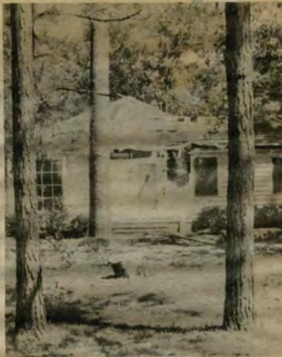
An unfortunate home-owner receives unexpected air-conditioning when Hurricane Elena knocks a tree through his front wall. (Photo by John Lambert, La. Military Newspapers)
