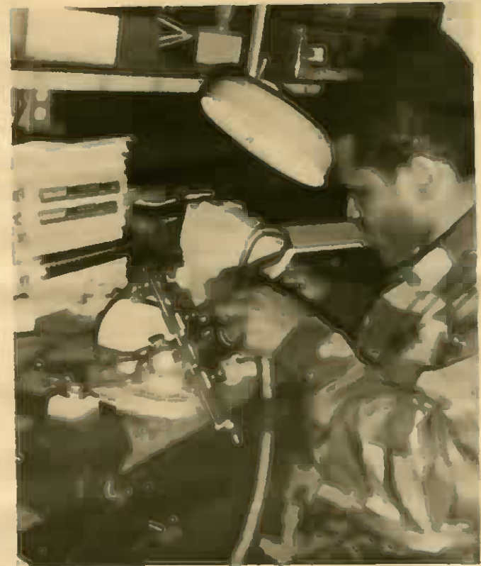
SSG Steven Francois solders cannon plug connectors for ground radio units. (Photo by TSGT David Eugene).
