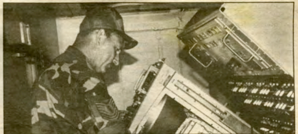
MSGT Nathan J. Lougue, air traffic control radar technician for the 236th Combat Communications Squadron, Louisiana Air National Guard, works inside the radar trailer of the Landing Control Central located in Hammond. (Photo by SPC Rebekah Lloyd-Smith, 241st PAD)
