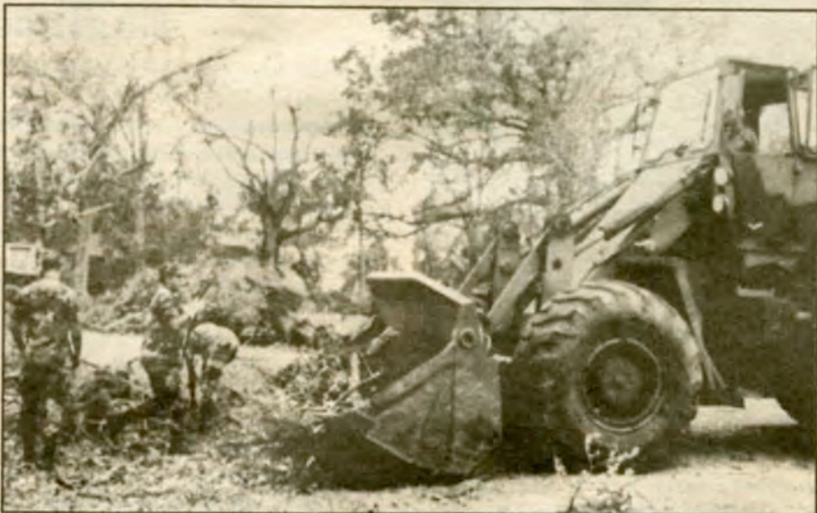
These engineers from the 769th and 527th Engineer Battalions (Cbt Hvy), 225th Engineer Group, Louisiana Army National Guard work together clearing First Street in Patterson, La., where debris collected after Hurricane Andrew. These engineers worked clearing impassable roads throughout southern Louisiana the night the devastating storm raped the state. (Photo by SGT Kristi
