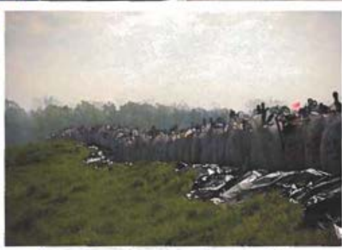
The two-mile line of super sacks stands as the only defense against the approaching flood waters of the Mississippi River.
