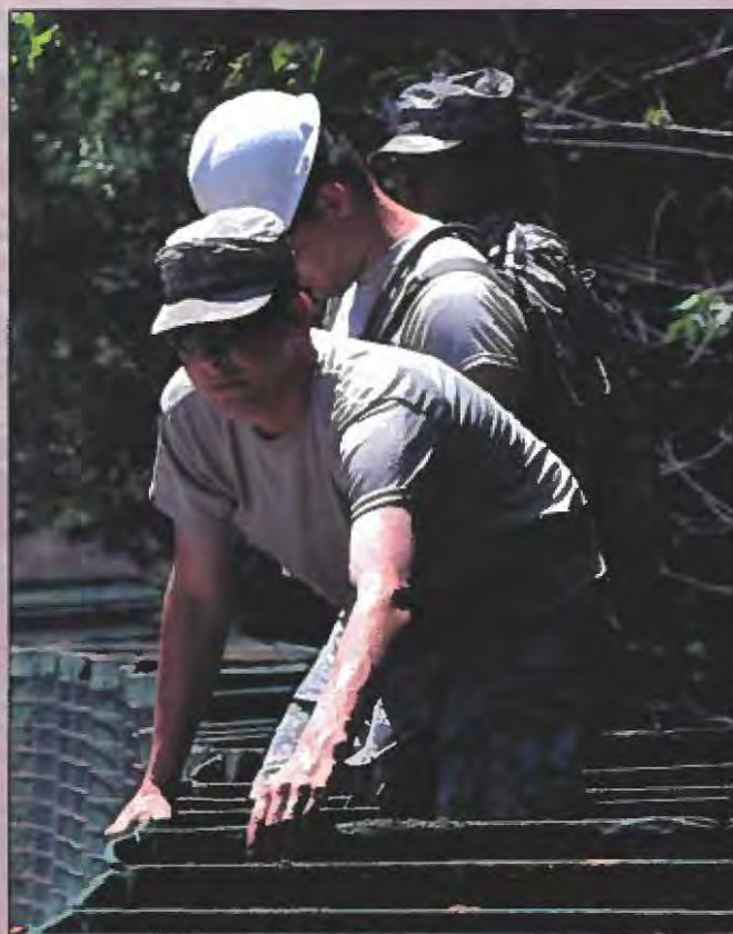
Pfc. Shelby Home and Spc. Eric Moos, both of the 769th Engineer Battalion, stretch HESCO baskets as part of a barrier project in Krotz Springs to protect a 240 home subdivision, a power substation and refinery, May 14, 2011. Photos: Master Sgt. Toby M. Velede
