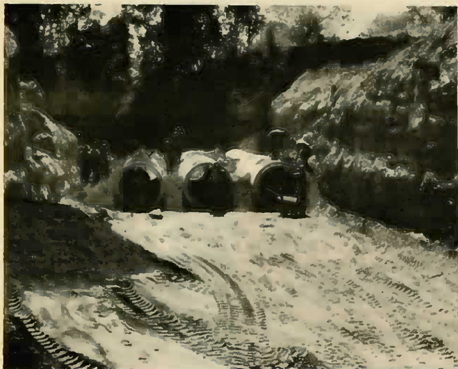
205th Engineers install culverts for the Triple -60. (Photo by CW2 Louis Joseph, 205th Engr Bn PAO)
