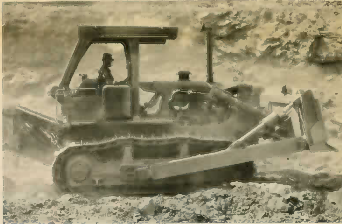
This soldier operates a D-7 dozer to clear rock debris off of the roadway.
