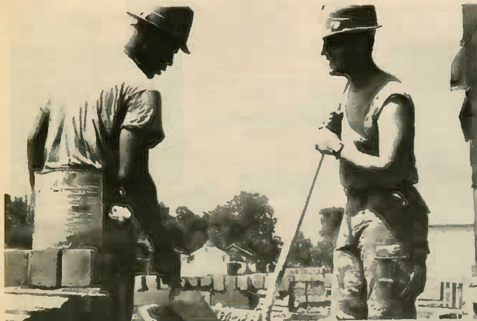
STIRRIN' THE BREW —PFC Steven Jupiter and SPC Charles Hicks stir mortar in a wheelbarrow. The mortar is used to hold the bricks in place that will be the foundation of an addition to the Louisiana State Military History and Weapons Museum. Jupiter and Hicks are part of the 528th's team that deployed to New Orleans for annual training. (Photo by SPC Mike Ritter, 241st PAD Staff)
