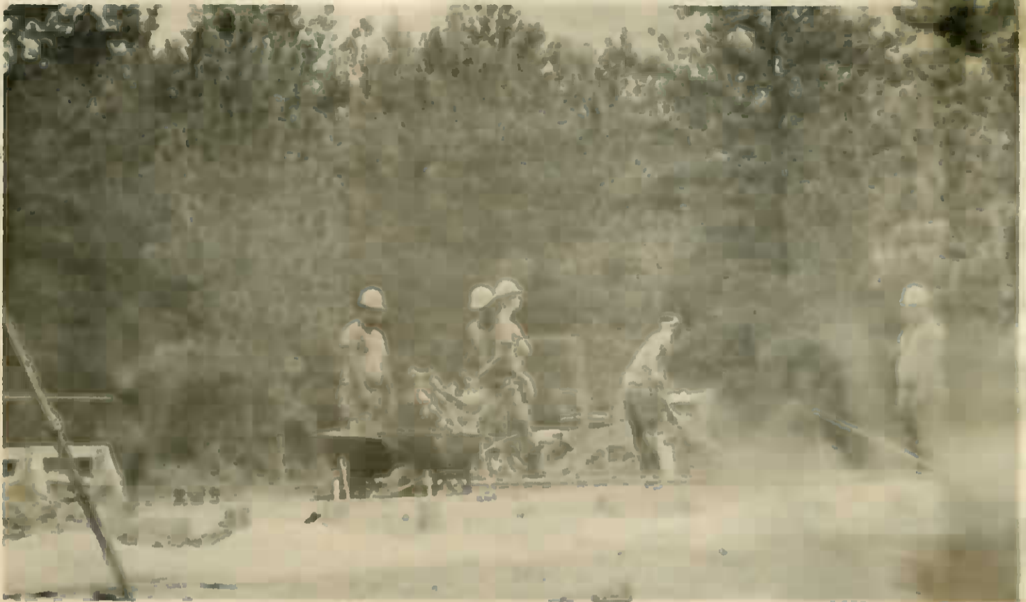
SPC Carlin Mills, SPC Donald Madison, PFC Jonathan Martin and SPC August Bennett backfill around the wooden forms, during annual training exercises 1991.
