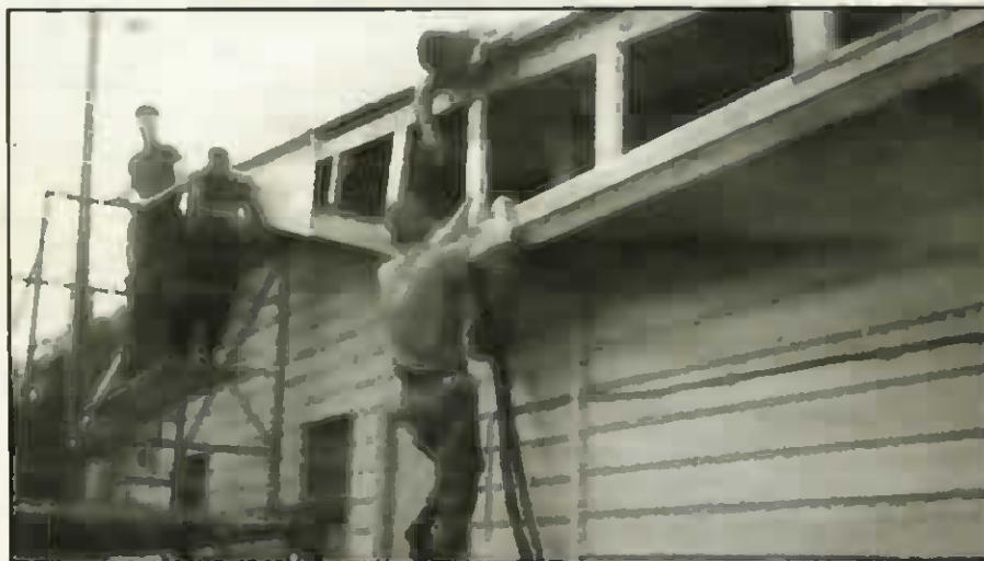
Members of 2nd Vertical Platoon, Company C, 769th Engr Bn install new rafters on the main building at VFW Post 3693 in Gonzales. (769th Photo)
