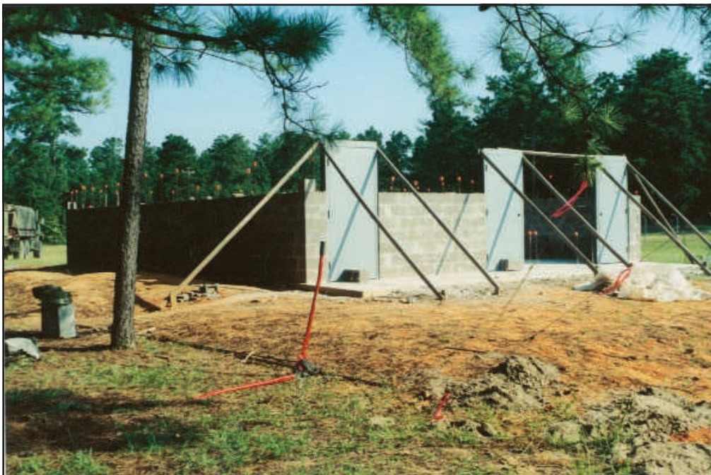
Cinderblock Latrine: During July, C Co, 769th Engr Bn worked on constructing a new cinderblock latrine at the Camp Beauregard Training Facility to replace an older wooden latrine. This latrine services the nearby Leadership Reaction Course. (Photo by MAJ Maria LoVasco, STARC PAO)
