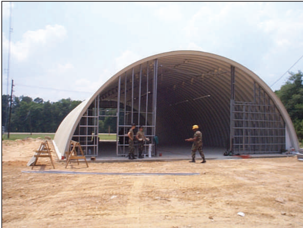
The 205th Engineer Battalion worked on several projects during Annual Training. They continued work on the two K-Spans at Camp Minden that will eventually house the HET Transportation unit. (Photo by MAJ Maria LoVasco, STARC PAO)
