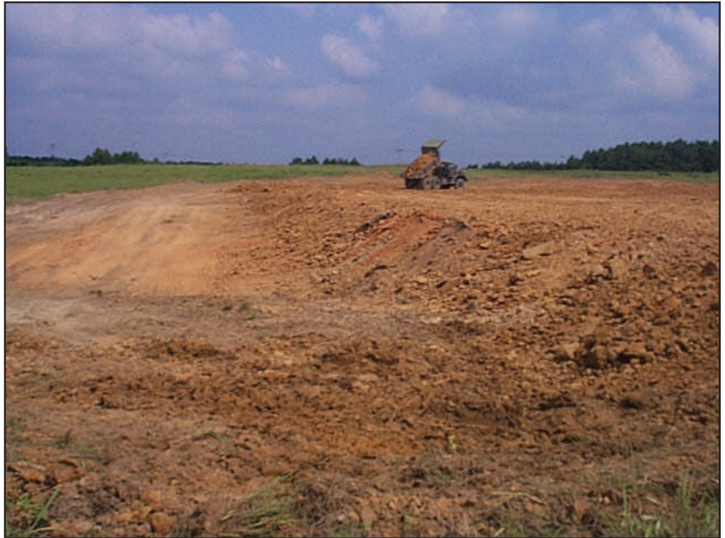
A dump truck releases a load of dirt into a gully being filled at the end of the runway at the Hart Memorial Airport in Many. Leveling the gully to the height of the runway will enable the runway to eventually be extended. (Photo by MAJ Maria LoVasco, STARC PAO)
