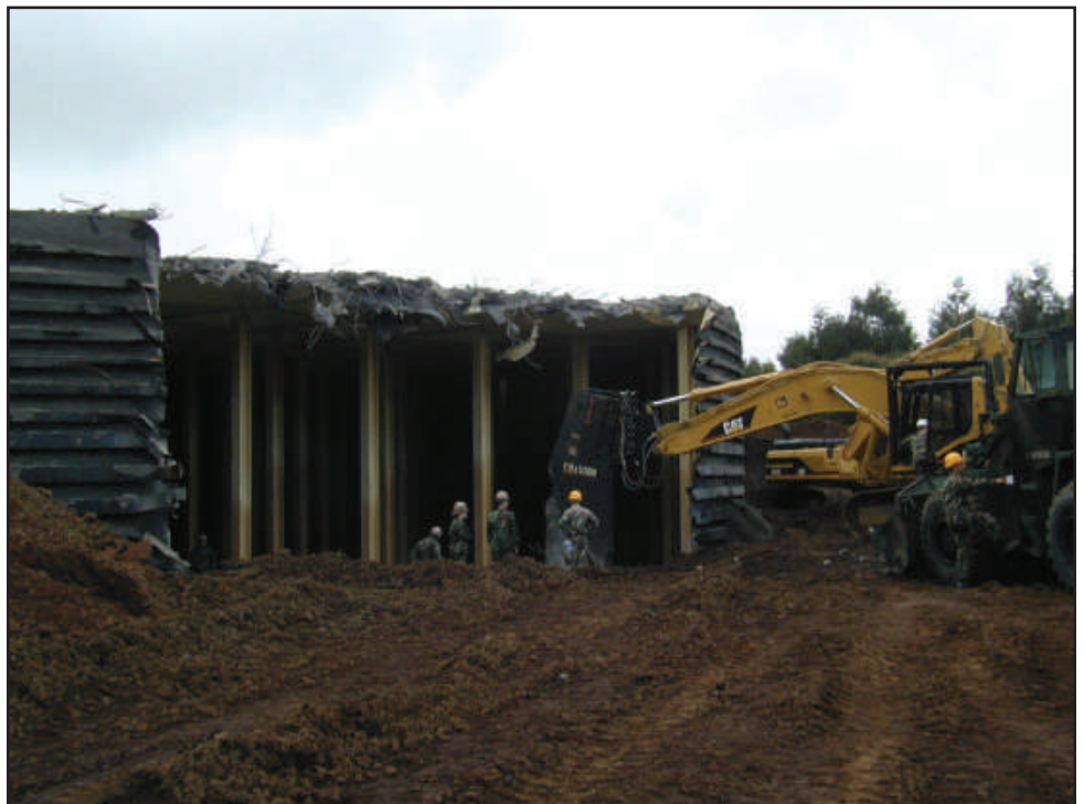
A Louisiana CAT excavator easily cuts through the reinforced steel and concrete fuel tank that sat abandoned at Lajes Field in the Azores. The 225 th deployed more than 100 Guardsmen this past summer to dismantle the tank at the request of the Portuguese government. (225 th Engr Gr Photo)
