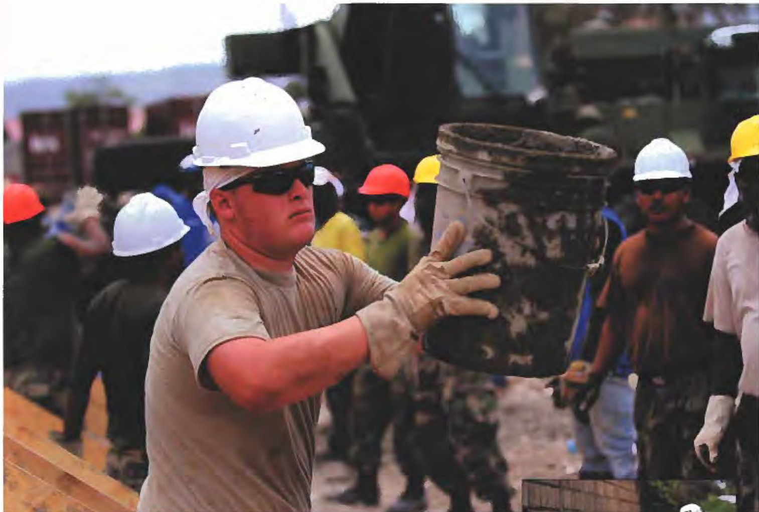
Spc. Jared Shelton of the Louisiana National Guard's 205th Engineer Battalion, 225th Engineer Brigade, works on the assembly line with Belize Defense Forces and local Haitian workers. The native of Sonama, La., passed five gallon buckets of mixed concrete July 14, 2010, to fill in the walls at the U.S. Army South New Horizons - Haiti 2010 Diaquoi school project in Gonaives.
