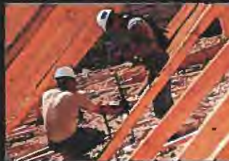
Soldiers of the 1021st Engineer Company, 205th Engineer Battalion, along with Belize military forces, prepare braces July 12, 2010, for school walls to be filled with concrete to construct a roof for the U.S. Army South New Horizons - Haiti 2010 Draqour School Project in Gonnaves.
