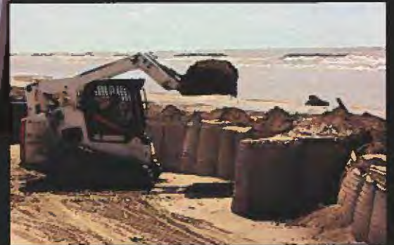
HOLLY BEACH, La. - Spc. Justin C. Boudin, 769th Engineer Battalion, 225th Engineer Brigade, fills Hesco baskets with sand along the coast of Holly Beach in Cameron Parish, La., July 14, 2010. Photo: Sgt. 1st Class Sara L. Piazza
